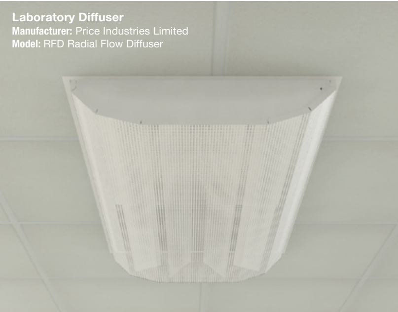
Laboratory Diffuser Manufacturer: Price Industries Limited Model: RFD Radial Flow Diffuser
